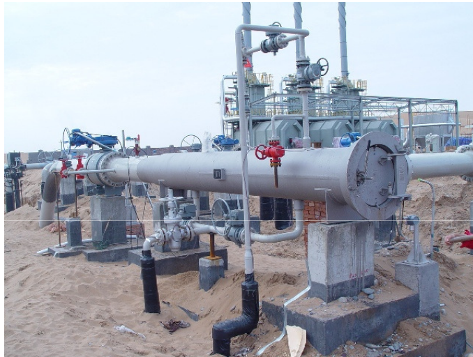
Typical Pig launcher/receiver installation.
